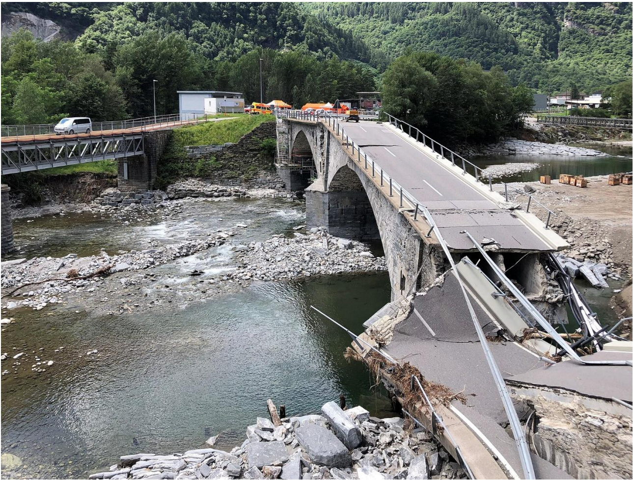
Figure 1- The collapsed Visletto bridge - source: Wikipedia ( https://de.wikipedia.org/wiki/Ponte_di_Visletto )
